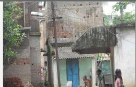
G+1 Houses catering to the needs of Beneficiaries (final stage)
