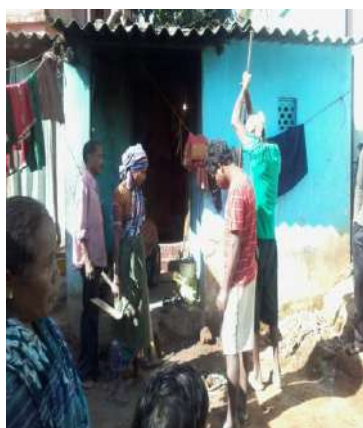
Water supply project in Slum
