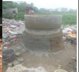
SHANTIPALLI DUSTBIN PIT
