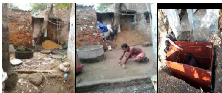
WELL REJUVENATION AND BATHROOM AT SHANTIPALLI
