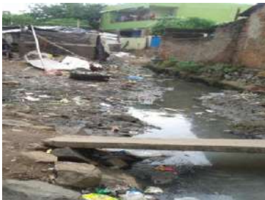
DRAIN RENOVATION AT KHAJA STREET
