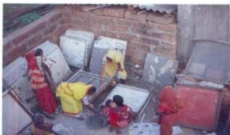
Mahila Milan members learning lady making for construction of low cost housing
